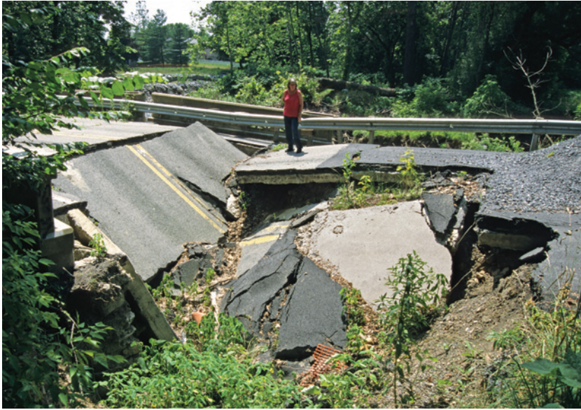
Fig. 11. A road in Pennsylvania destroyed when it dropped into a new subsidence sinkhole that had been largely induced by drainage of a deep quarry more than a kilometre away.
